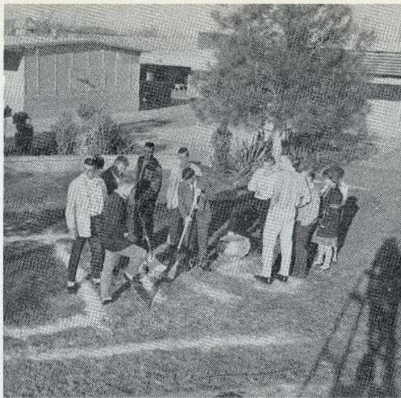
Cleanup under way
