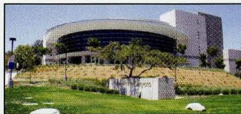
The College of the Canyons Performing Arts Center features a 926-seat main theater and the smaller Black Box Theater, which seats up to 125 people.
