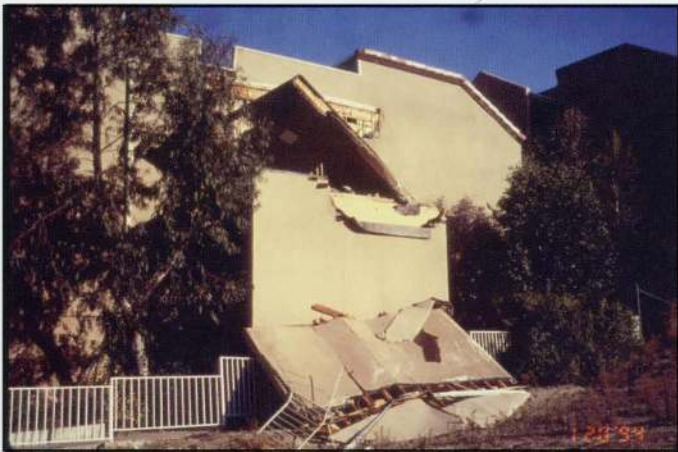
Buildings, homes, roads, walls and bridges collapsed as a result of the 1994 Northridge earthquake that rocked Santa Clarita Valley.
