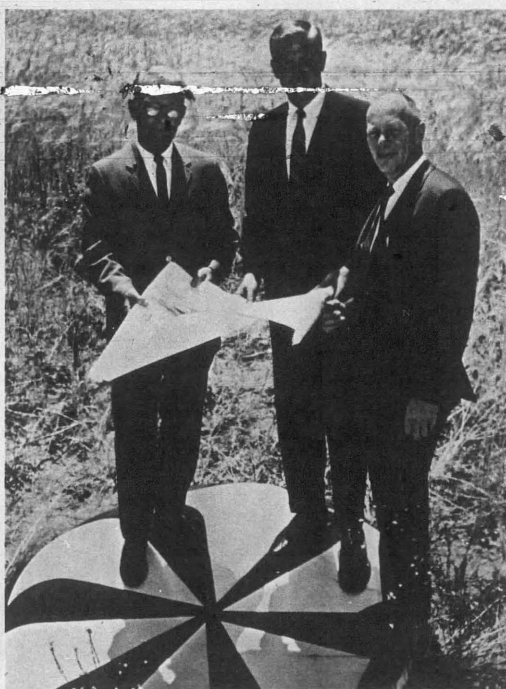
The Rotella marks the spot where construction began on the new M. W. Sausse plant in Valencia Industrial Center. Company president, M. W. Sausse (left), Caland vice president, Peter Kremer (center) and Architect William Reidenbach (right) watch earth moving equipment move into position to begin work on the building planned for completion September 30. The Sausse Company is a leader in vibration control equipment.
