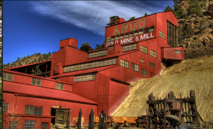
Argo Tunnel and Mill, Clear Creek County, CO Thad Roan
