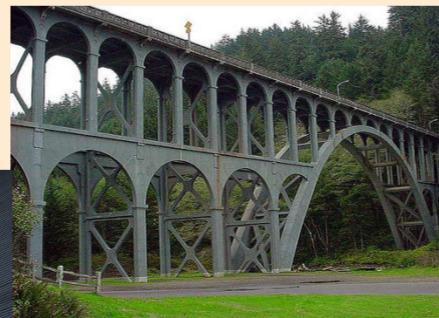
Cape Creek Bridge No. 01113 Lane County, OR Bruce Fingerhood
