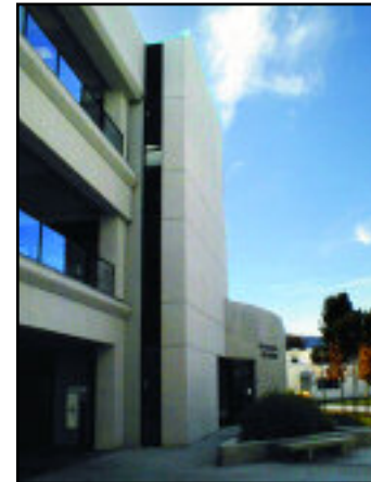
The steel framework (top) is pieced together to create the Media & Fine Arts Building (above).
