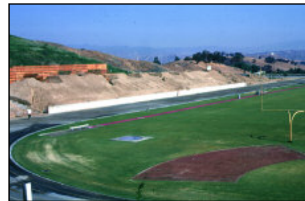
A crane hoists a bank of lights into place at Cougar Stadium, which itself is under construction (top). An earlier photo (above) shows the field, running track and a mound of dirt that was used as the foundation for the stadium.
