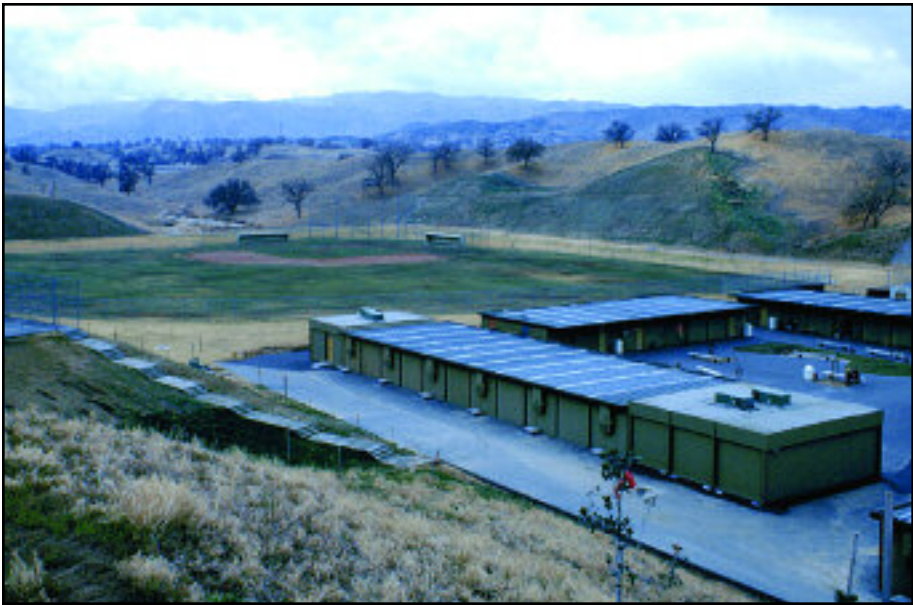
The first campus at the permanent site was composed of a collection of temporary modular buildings holding 99 classrooms. The buildings of the so-called "instant campus" sat roughly on the location of the present-day softball field.
