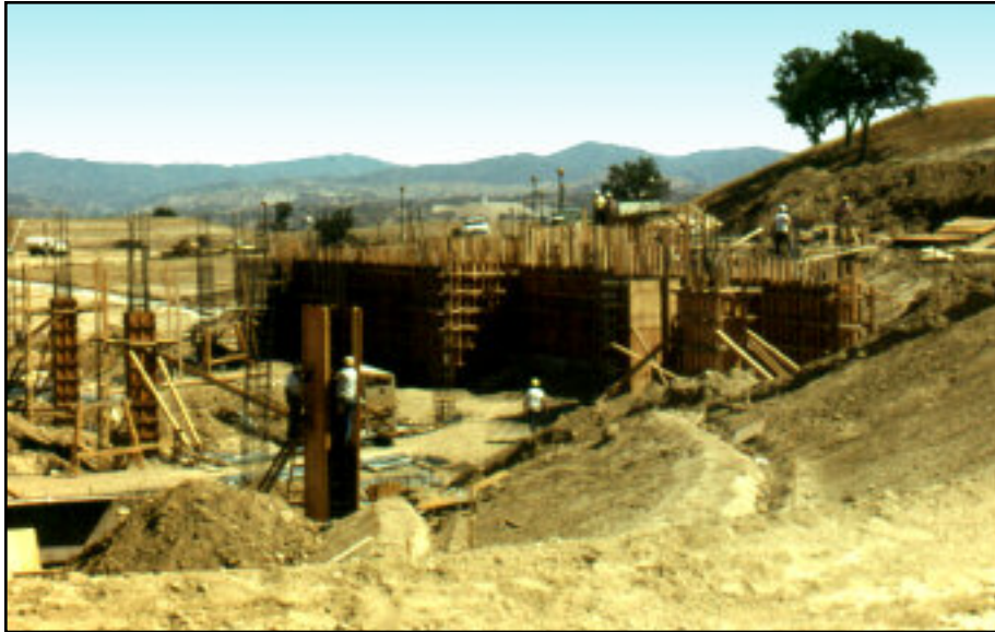
Construction workers build the forms that will encase the massive poured-concrete foundation of the Instructional Resource Center.
