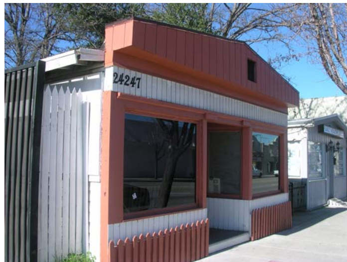
Tom Mix Cottage 1, 24247 San Fernando Road
