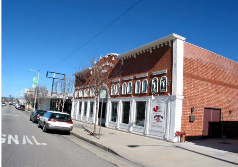
The Canyon Theater Guild Building 24242 San Fernando Road built in 1948 and extensively renovated. View to northeast of Canyon Theater Guild Building west façade and south elevation.
