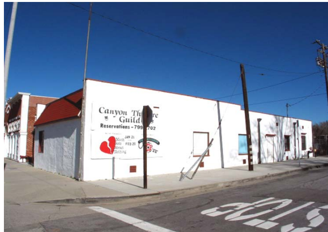
When compared to the above historic image, this January 2005 view of the south elevation and west façade indicates that a door and window have been removed from the façade.
