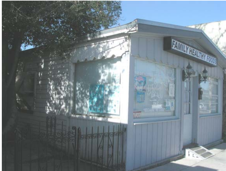
Tom Mix Cottage 2, 24251 San Fernando Road
