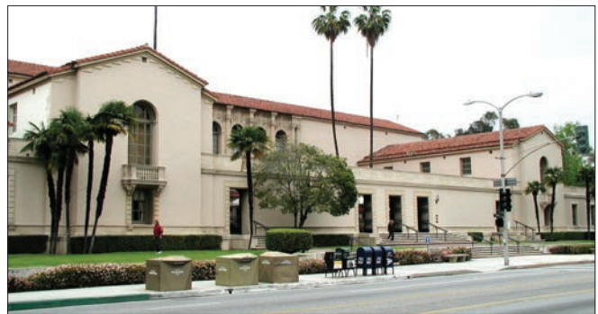
A public building addressing one street and terminating another with a forecourt
