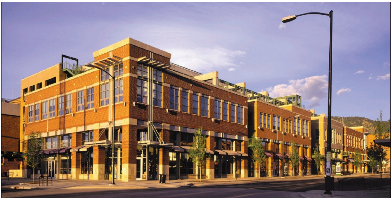
Park Once Garage (in Boulder, CO)
