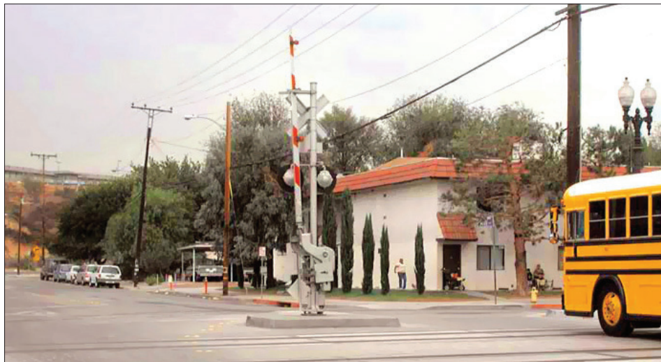
Overhead utilities on Market Street at Pine Street
