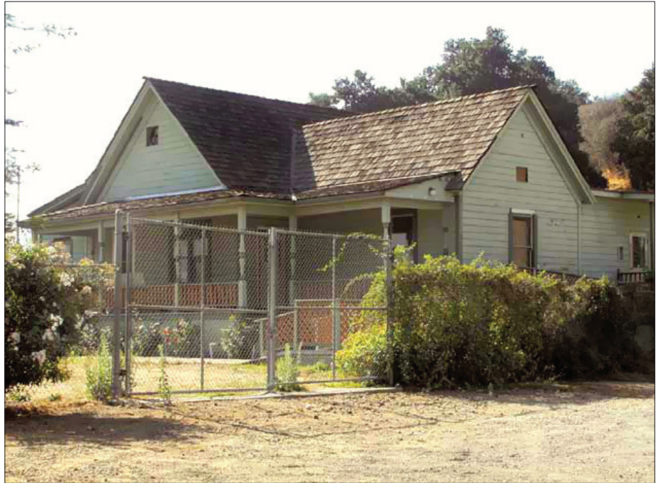
A. Visitor's Center: Historic Pardee House to be relocated at south entry to Old Town Newhall
