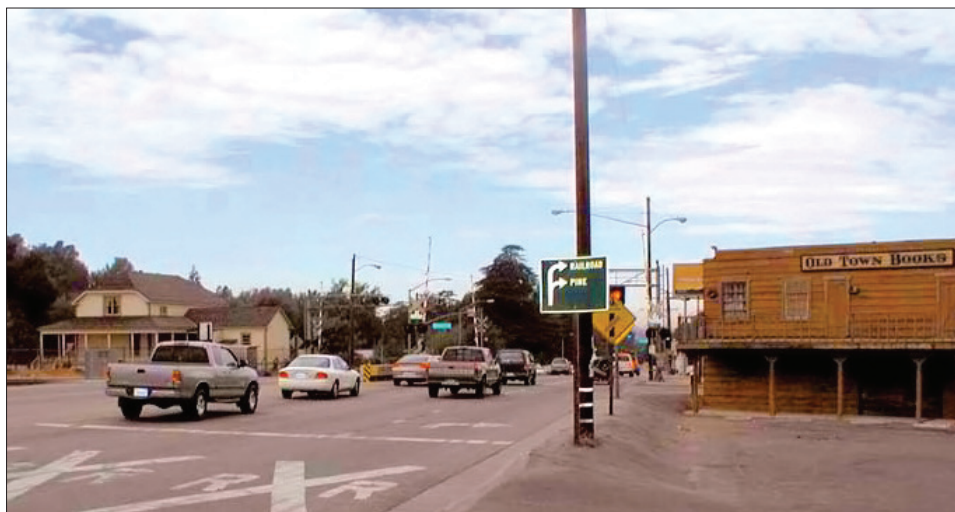
Overhead utilities at south entry to Old Town Newhall
