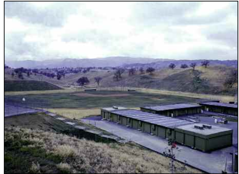
The first campus at the permanent site was composed of a collection of temporary modular buildings holding 99 classrooms. The buildings of the so-called "instant campus" sat roughly on the location of the present-day softball field.
