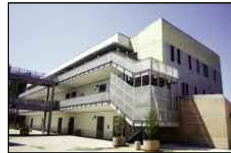
Newly built Aliso Hall (top, right) is clustered with the existing science building, Boykin Hall (top, left), and Aliso Labs (above).
