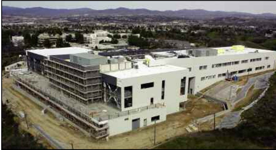
The University Center takes shape in this low-aerial view looking northeast in February 2009.
