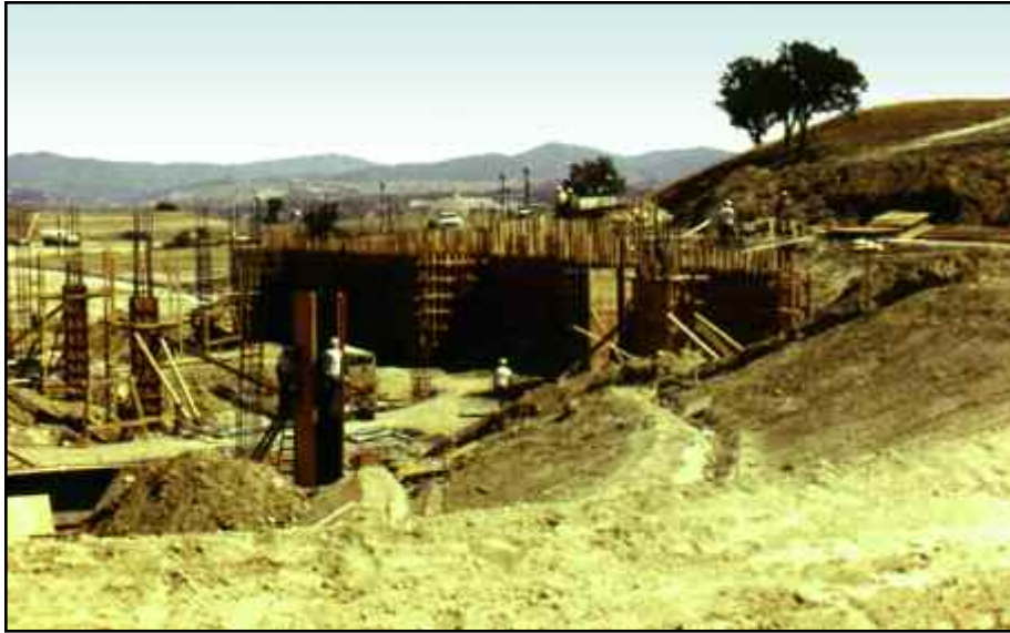
Construction workers build the forms that will encase the massive poured-concrete foundation of the Instructional Resource Center (Bonelli Hall).
