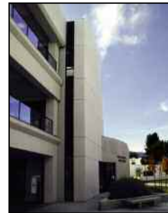
The steel framework (top) is pieced together to create the Media & Fine Arts Building (Mentry Hall, above).
