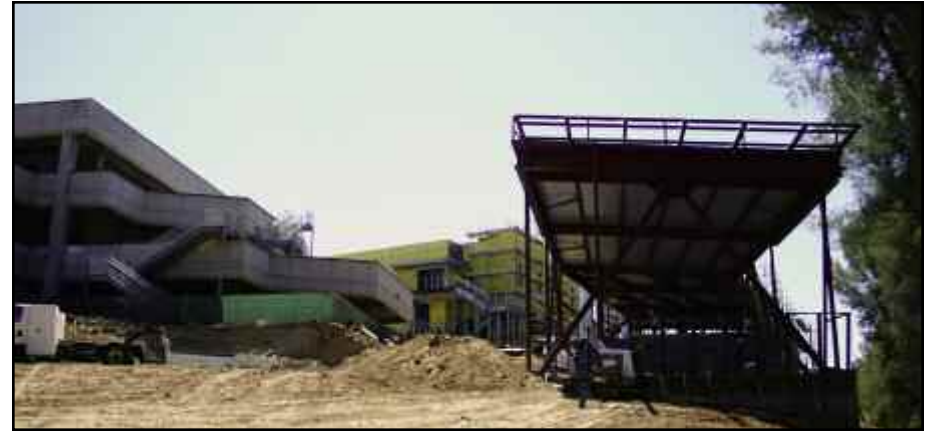
Construction of Aliso Hall (above, right) and Aliso Labs (above, center) moves forward adjacent to Boykin Hall (above, left) in mid-2006.
