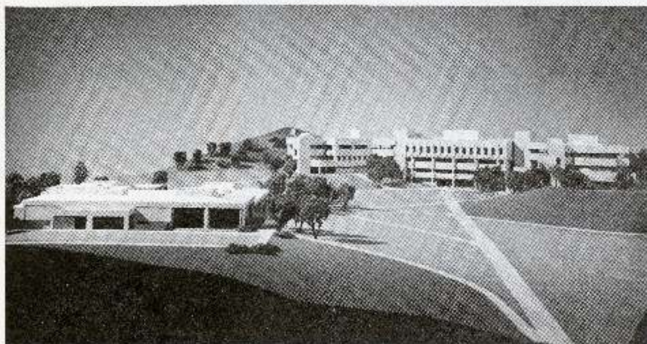
First building expected to be constructed on campus is the Instructional Resource Center (see story below). Walkway at right in photo leads to the IRC building. If state funds are released next week as expected, IRC groundbreaking ceremonies will be held in mid-April, and the building will be ready for occupancy for the 1973 fall term.
