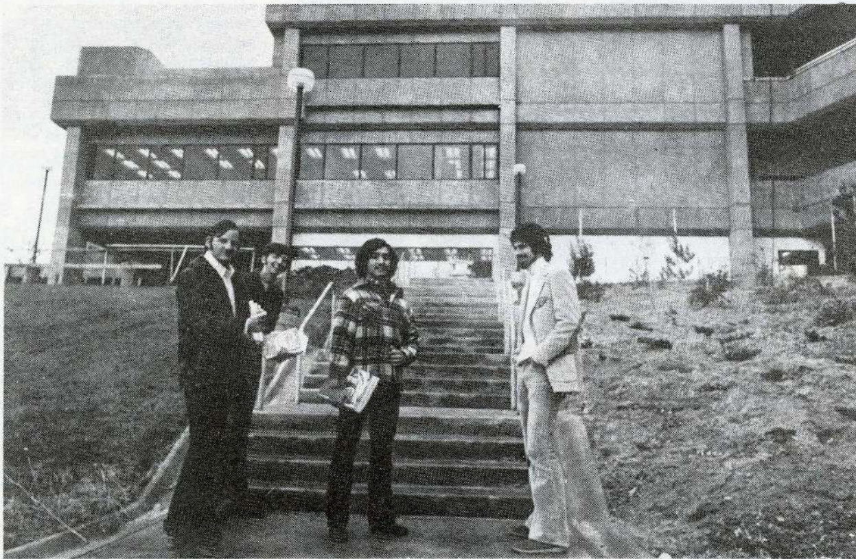
The Classroom Center, the third major structure to be constructed at COC, will be occupied this week by departments still on the lower campus. Pictured (from left) are Scott Taylor, John Crnkovich, Jina Aceves and Michael Shannon. The center, which costs $950,000, contains offices for administrators and space for an ultimate computer center as well as classrooms. Next building to be occupied is the Student Activities Center which should be partially ready next month.
