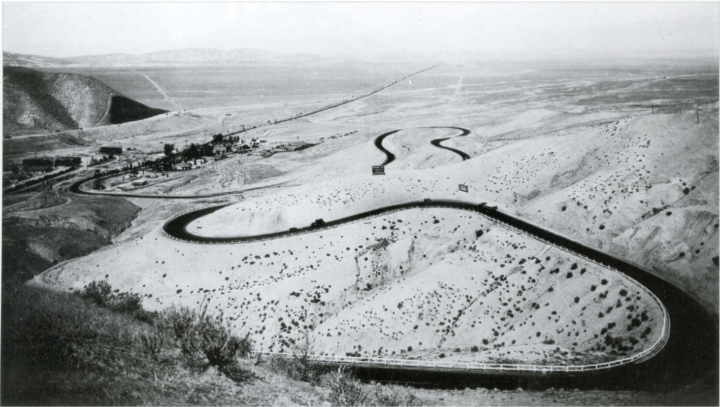
The steep grade and many switchbacks of the Grapevine made it one of the most treacherous spots on the Ridge Route for many truckers.
