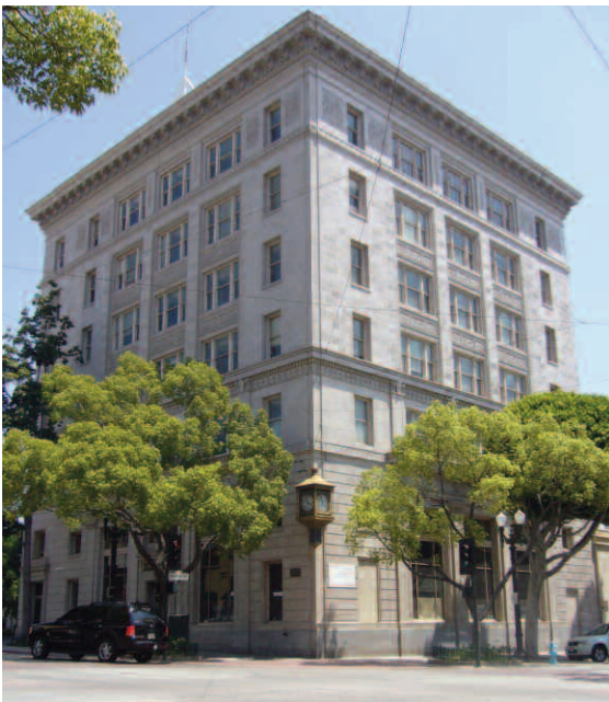
Whittier's historic preservation ordinance does not require owner consent for the designation of local landmarks, increasing its effectiveness as a tool for protecting the city's architectural heritage. Pictured above: National Bank of Whittier (1923), Whittier Historic Resource. Photo by Conservancy staff.
