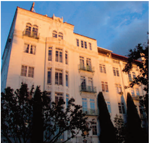
Top: Self Help Graphics & Art Building (1927), unincorporated East Los Angeles, Los Angeles County (Conservancy staff)
