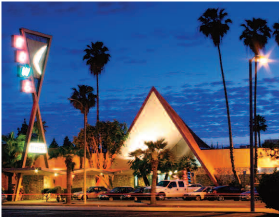
Top: South Seas House (1902), West Adams, Los Angeles Historic-Cultural Monument No. 757 (West Adams Heritage Association)
