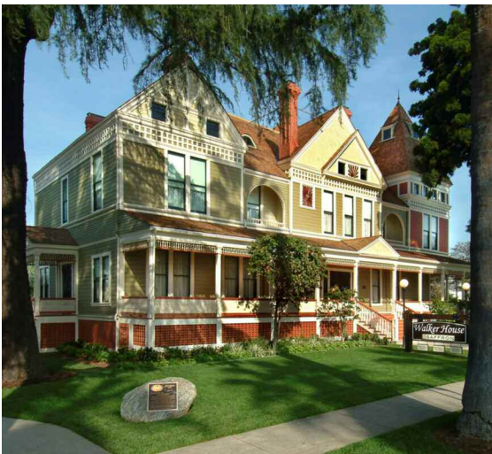
The City of San Dimas led the effort to restore and rehabilitate the Walker House (c. 1887), earning a Los Angeles Conservancy Preservation Award in 2010. Photo by Pete Bleyer.
