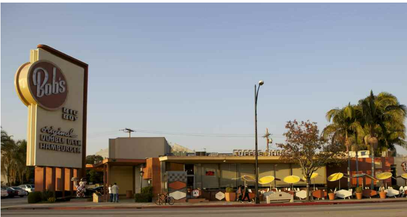
Bob's Big Boy (1949) in Burbank, a beloved community gathering place that was once threatened with demolition. Photo by Holly Hayes on Flickr.
