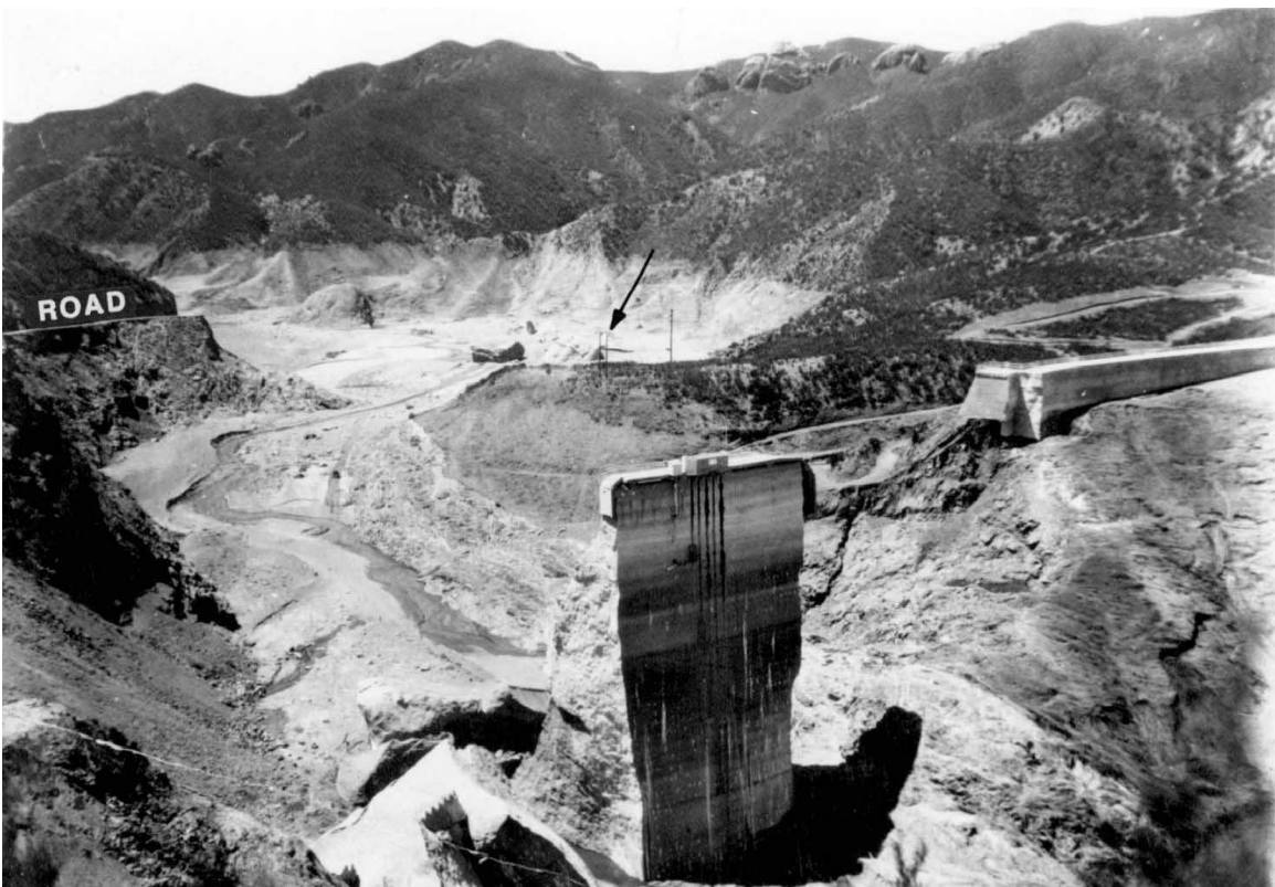
Figure 16. Downstream view after dam failure, showing standing block No. 1, a portion of the western wing dike, and scour line of the flood waters. Date unknown. (Ventura County Museum of History and Art, with notations by Rogers)
