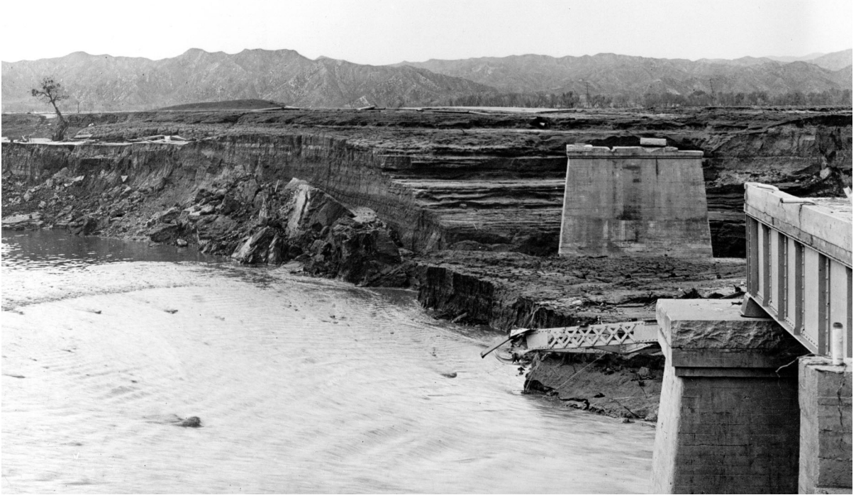
Figure 7. The remains of a highway bridge crossing the Santa Clara River near Castaic, probably photographed with a week after the dam's collapse. (John Nichols Collection)
