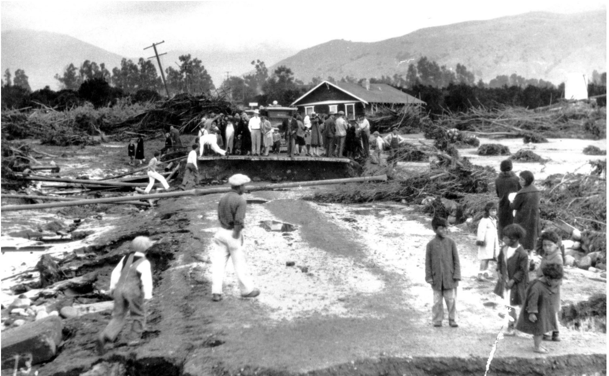
Figure 8. Santa Clara Valley residents inspecting a road washout on the northern approach to the Bardsdale Bridge, near Fillmore, probably on March 13, 1928. (John Nichols Collection)
