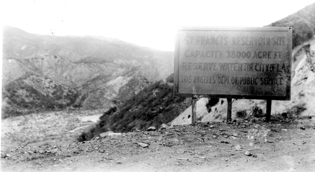
Figure 1. Sign advertising the construction of the St. Francis Reservoir, probably taken from the dam road on the south side of San Francisquito Canyon in late 1925, after the dam's storage capacity was raised to 38,168 acre feet. (United Water Conservation District/John Nichols Collection)
