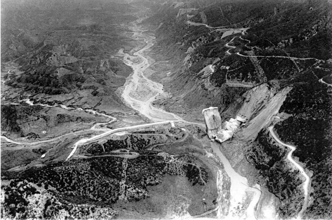
Figure 15. Aerial oblique upstream view toward the north/northeast at the dam site on March 13, 1928. Standing block No. 1 is visible in the center right middle ground, and the remaining sections of the wing dike on the dam's western abutment on the hillside to its left, as well as the massive landslide on the dam's eastern abutment. (Spence Collection, UCLA Dept. of Geography)
