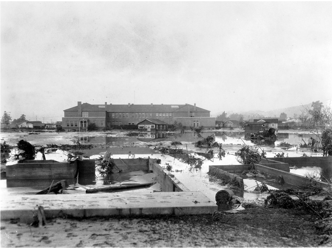
Figure 11. The Isbell Middle School in Santa Paula, and the foundations of the homes previously located on nearby streets, one of which is seen dislocated into the school yard. Photograph probably taken on March 13, 1928. (John Nichols Collection)
