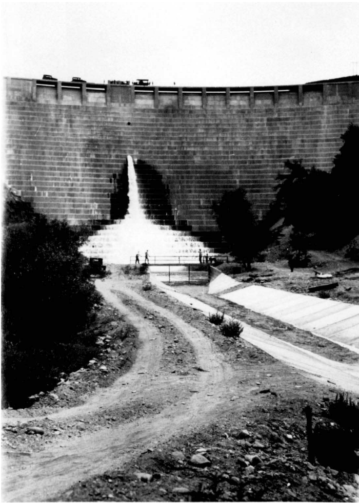
Figure 3. Downstream view of the face of the St. Francis Dam after its completion. The only day water was known to have been released from the reservoir into San Francisquito Creek after the construction of the dam began in 1924 was on the day it failed, but this photo was probably not taken on March 12, 1928. (Los Angeles Department of Water and Power)
