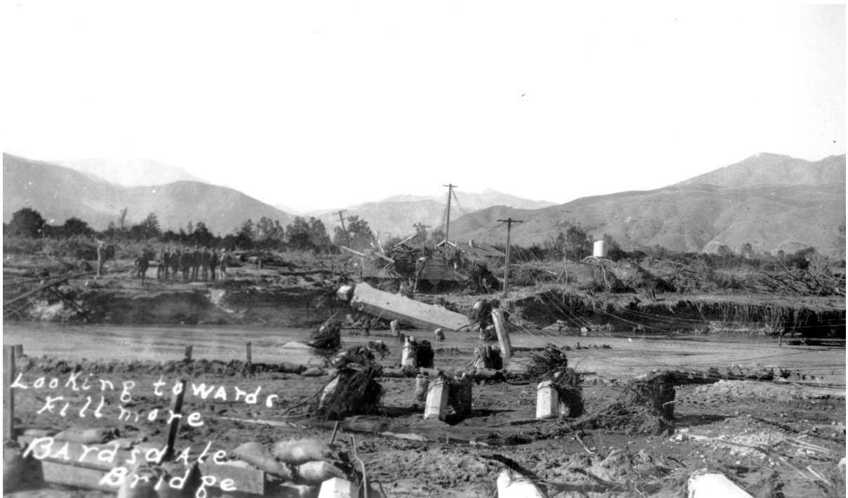
Figure 9. The remains of the Bardsdale Bridge, probably as photographed within a week of the dam's collapse. (John Nichols Collection)
