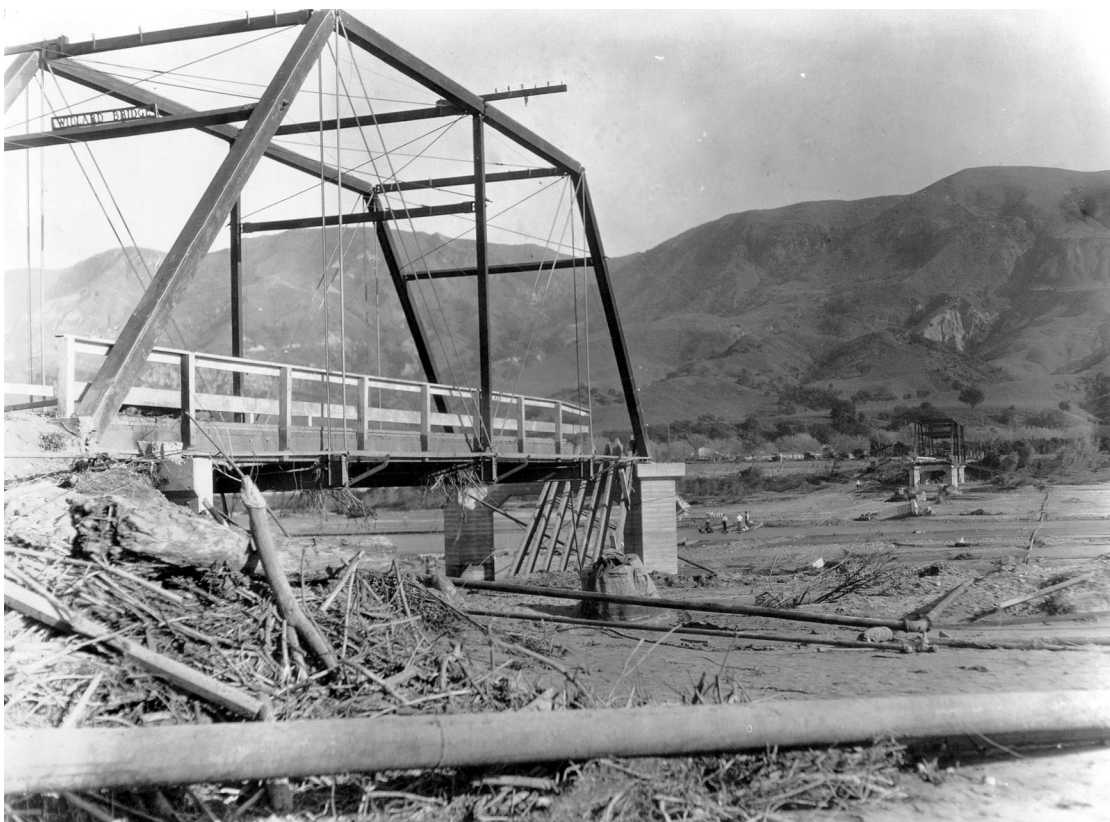
Figure 10. The Willard Bridge, east of Santa Paula, destroyed at 3:00 AM on March 13. Photograph probably taken within a week of the dam's collapse. (John Nichols Collection)
