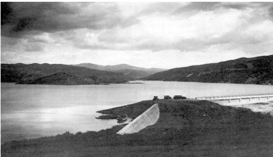
Figure 4. Portion of a panorama photo of the completed St. Francis Reservoir facing southeast, with the dam's western wing dike visible in the right middle ground. This photo was probably taken in early March 1928. (Los Angeles Department of Water and Power)
