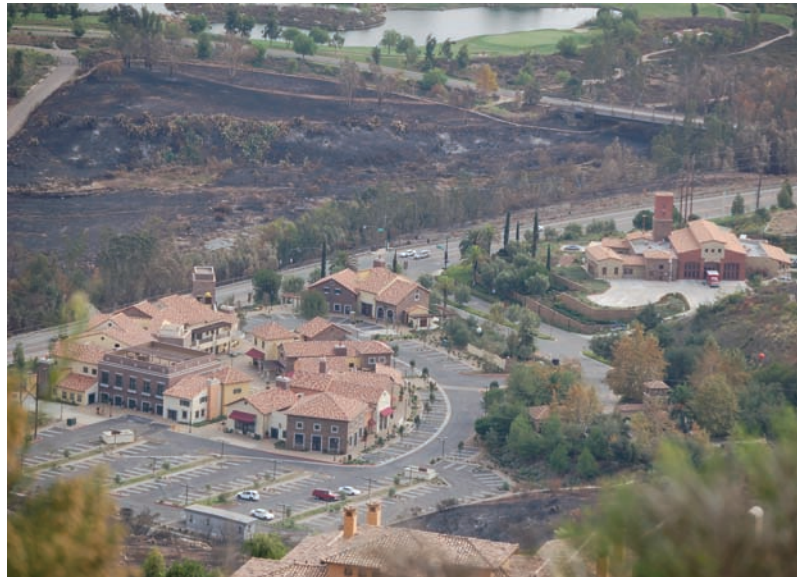
Many communities built with fire safe building practices passed the ultimate test by surviving the siege.
