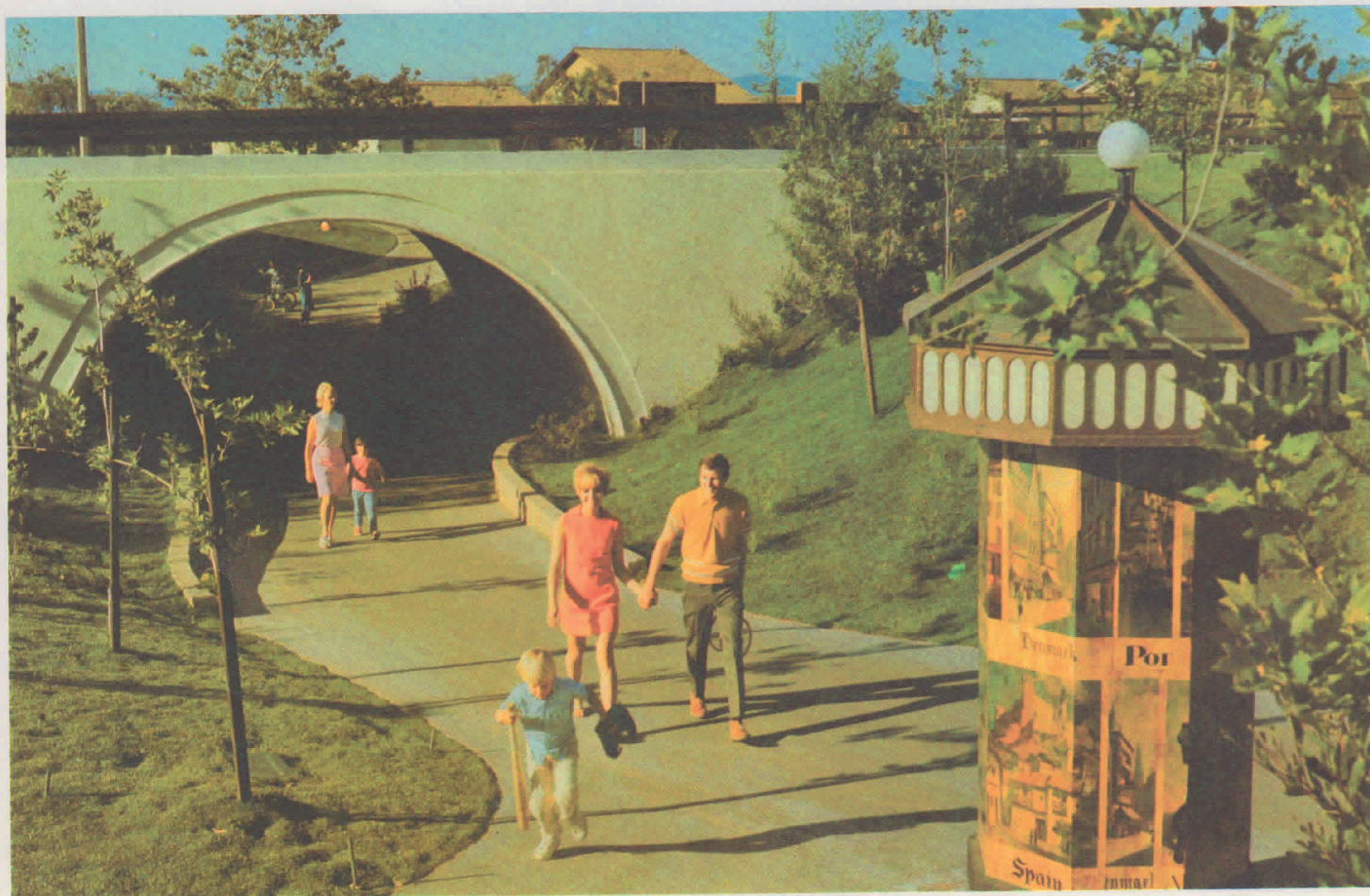
The beauty of underpasses... safety.
