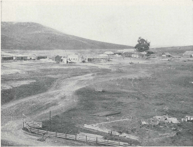
Site of the present Richmond Refinery on San Francisco Bay, photographed in 1901, when construction work began. Here the Standard Oil Company erected the then largest single refinery in the world and connected it by pipe-line with the distant oil-fields in the San Joaquin Valley
