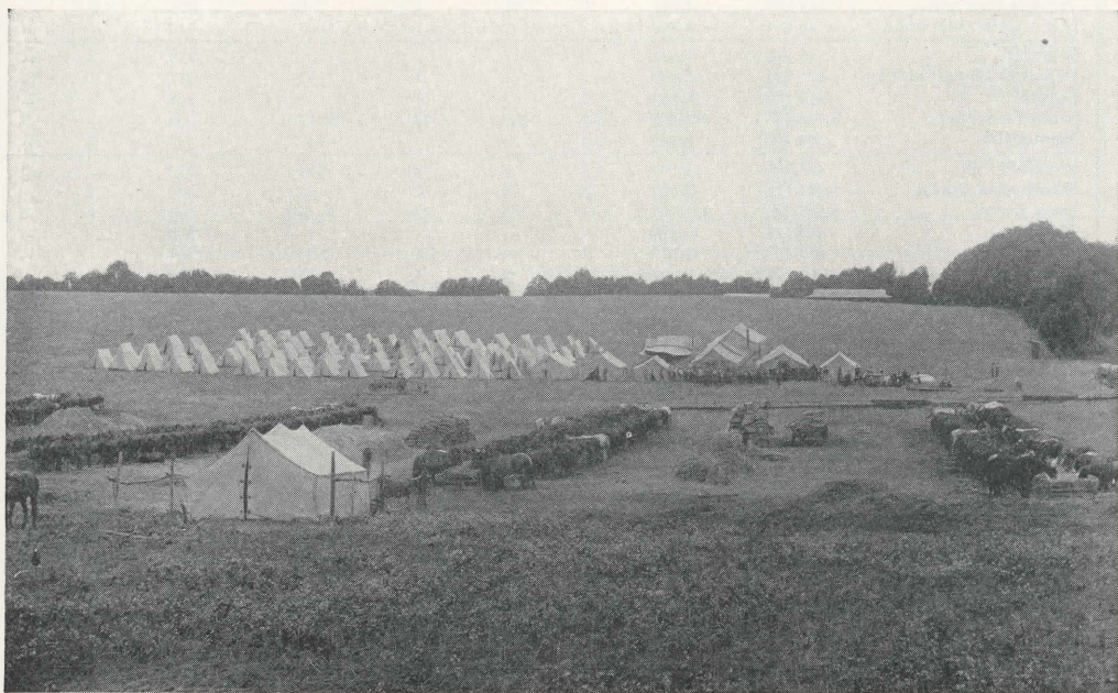
When it became apparent that there was likely to be sufficient crude-oil production "south of the Tehachapi" to warrant a refinery in southern California, the Company decided to construct one. Above photograph depicts the camp on the site of El Segundo Refinery the day before the first ground was broken for still foundations. More than five hundred mules are feeding
