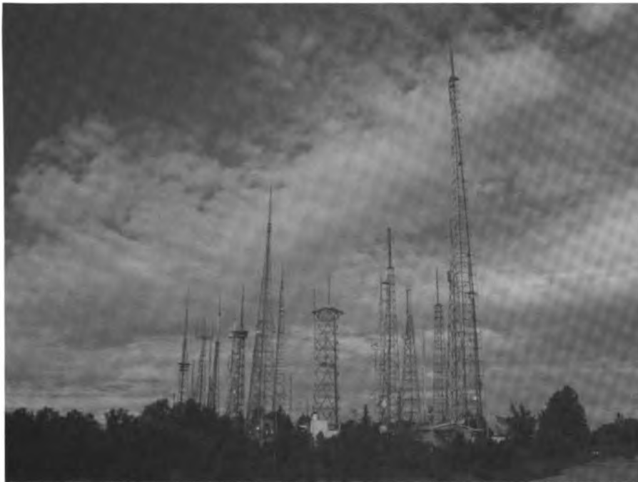
Mt. Wilson Telecommunications Site
