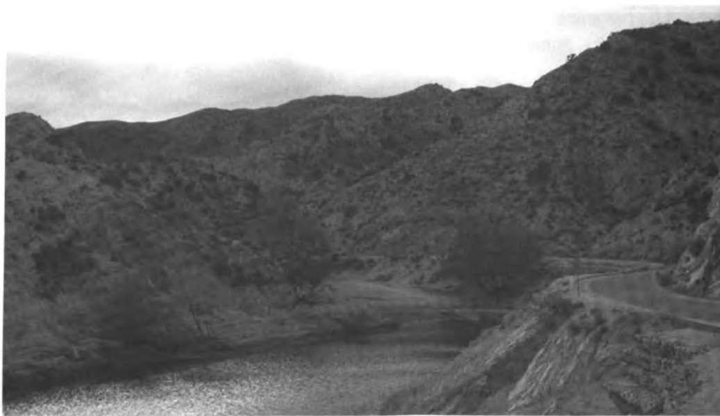
Little Rock Dam
